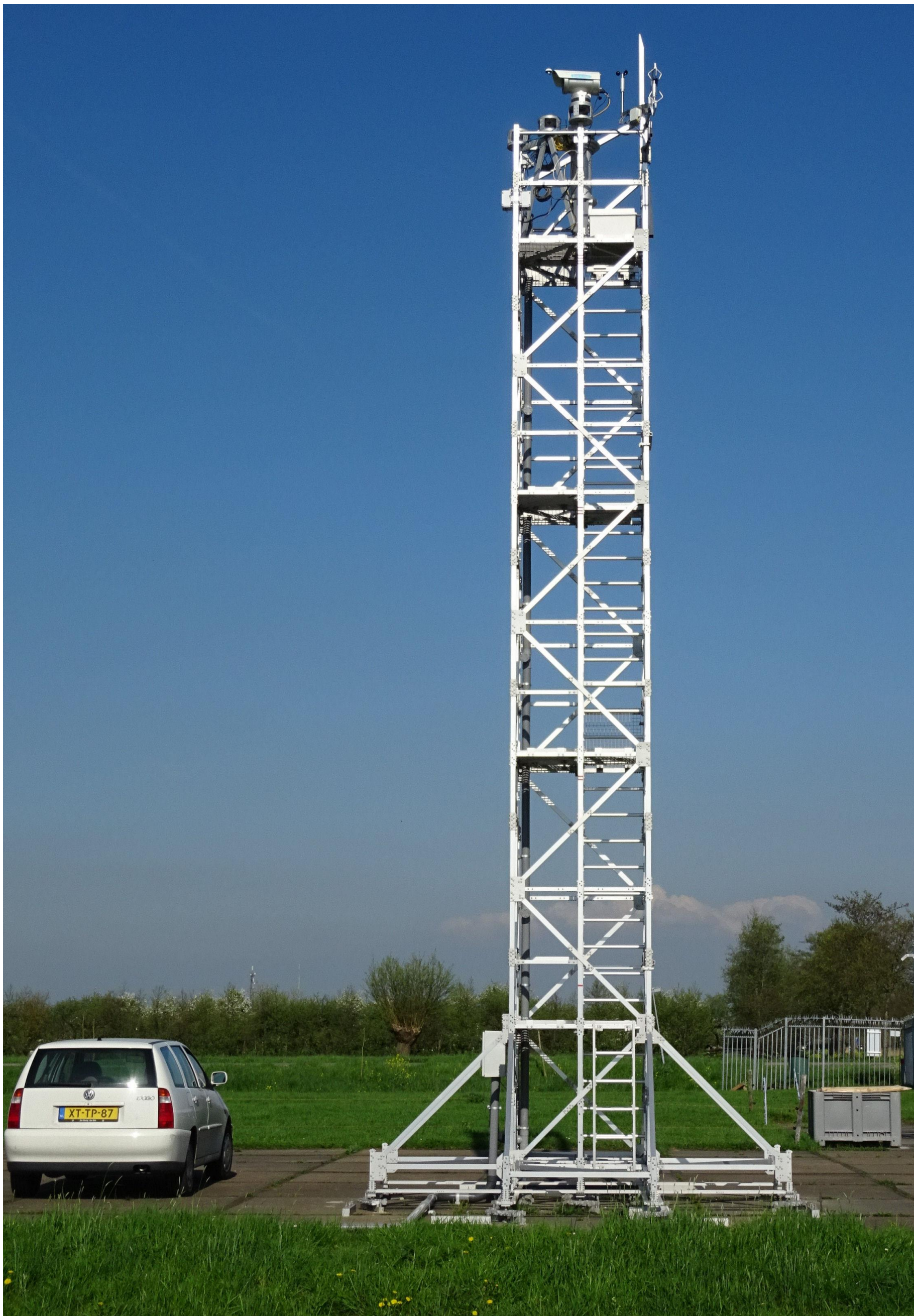
Figure 4. Second tower with on top the LAS Receiver, like the Transmitter a 15cm aperture telescope, which is precisely pointed to the Transmitter on the first tower at the left side on 900m distance. Wind is measured by cups for velocity and vane for direction and also by a 3-D ultrasonic acoustic anemometer, which sticks outside the top platform and is shown in detail in Figure 5. It is able to measure very fast the wind speed and direction.
