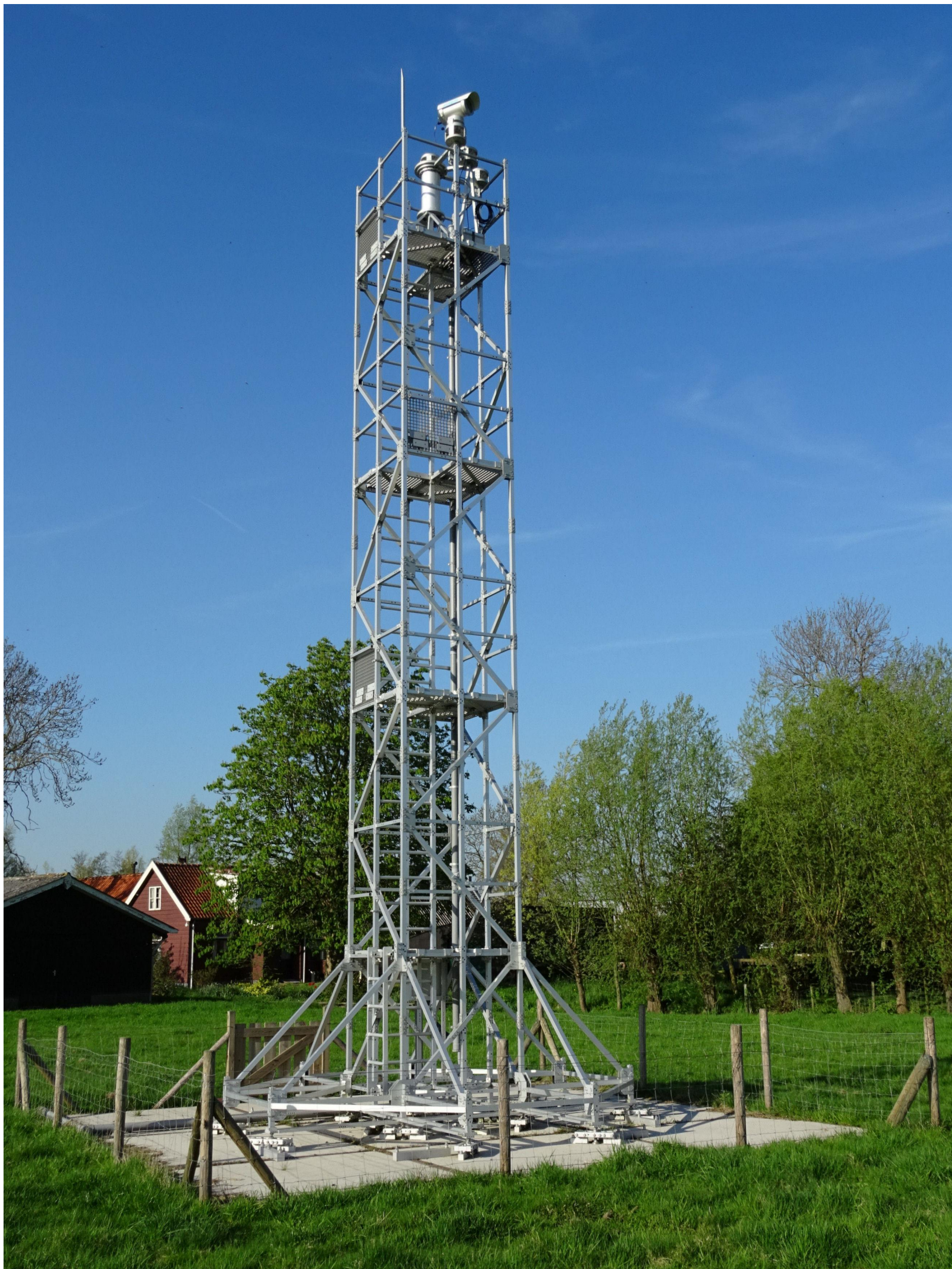
Figure 2. First tower with on top the Transmitter of the Large Aperture Scintillometer (LAS), the 15cm aperture telescope pointed in the right front direction exactly to the Receiver on the second tower on a distance of 900m. This photo is made before all the additional instruments were installed. It shows how the Transmitter is mounted on the top of the tower. The peak gives protection to the transmitter against lightning.
