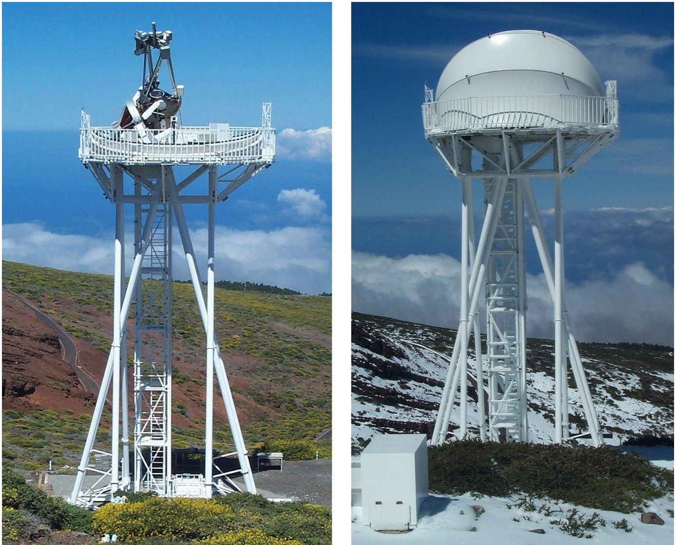
Figure 2. The DOT on its open steel framework tower with a height of 15m. The left picture shows the enclosure open while the DOT is observing. The right picture shows the enclosure closed as protection against bad weather. A framework is around the ladder with every 2.5m a platform, where the climbing side changes. Consequently, fall height inside the framework at maximum 2.5m and safe climbing without safety belt.
