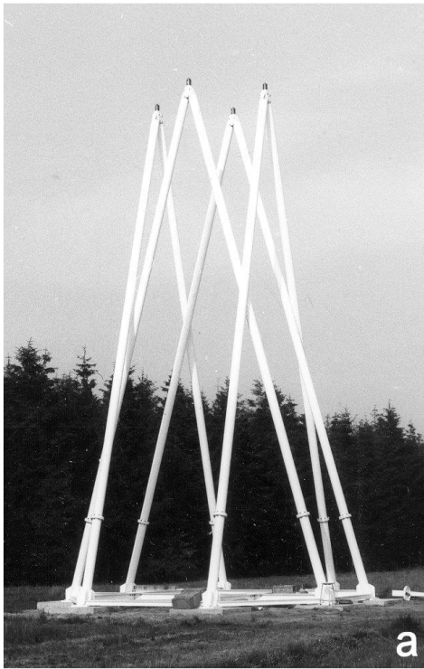
Test assembly of the inner platform on the 4 triangles in Westerbork a. 4 triangles assembled b. the tops of the triangles c. the inner platform is hoisted to the triangle tops
