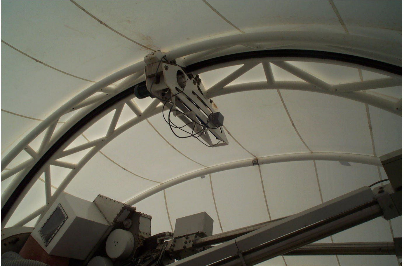
Figure 14. The textile membranes seen from the inside of the closed dome. The membranes are curved to the inside of the dome from bow to bow, and curved to the outside going from one dome side with downward bow ends to the other side of the dome with downward bow ends. This two sided curvature in opposite direction is similar to the shape of a saddle, so this membrane shape is called saddle shape. Consequently, the membranes are not flat pieces of textile. If one tries to put a membrane on a flat floor, then the rims are longer than the centerline along the membrane, and hence, the rims lie in waves.
