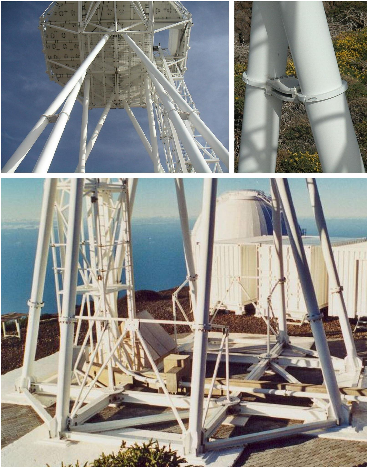
Figure 11. Vibrations caused by wind, known as Vortex Oscillations and explained in Table 1 , are reliably prevented with dampers between the tubes. Figure 2 left side shows, that, for all tubes, two tubes pass closely to each other at half tower height. There, dampers are placed between the tubes. Top left: The dampers seen from the base of the tower. The damper on the right is near the ladder. Top right: Damper in close up seen from the ladder. Two flexible rubber plates connect the tubes. The drawing in Figure 11a shows the parts of the damper construction with dimensions. Bottom: From each pair of tubes with damper in between, the free length of one tube is shortened with additional small tubes perpendicular to the upward tube at a height of 2.34m, bringing the resonance frequency from 5.8Hz (see Figure 8 ) to about 7 Hz. Consequently, the two upward tubes with damper in between can not vibrate together, giving reliable prevention of vibrations. The small perpendicular tubes do not disturb the compensation principle for parallel motion of the platform.
