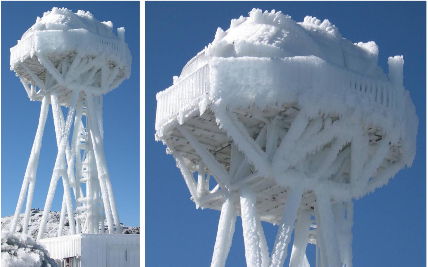
Figure 13. Extreme weather situation to which the completely open-foldable is able to protect the telescope. Intense ice growth has taken place during the stay in a supercooled cloud. However practically no ice sticks on the textile membranes, whereas there are huge amounts of ice on all metal parts, like the bows, which are strong enough to withstand the heavy ice load.
