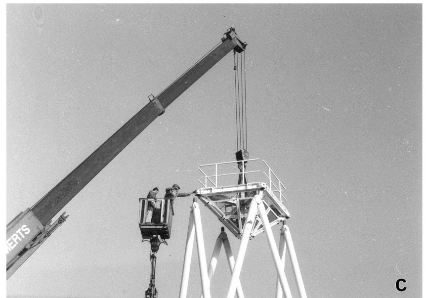
Test assembly of the inner platform on the 4 triangles in Westerbork a. 4 triangles assembled b. the tops of the triangles c. the inner platform is hoisted to the triangle tops
