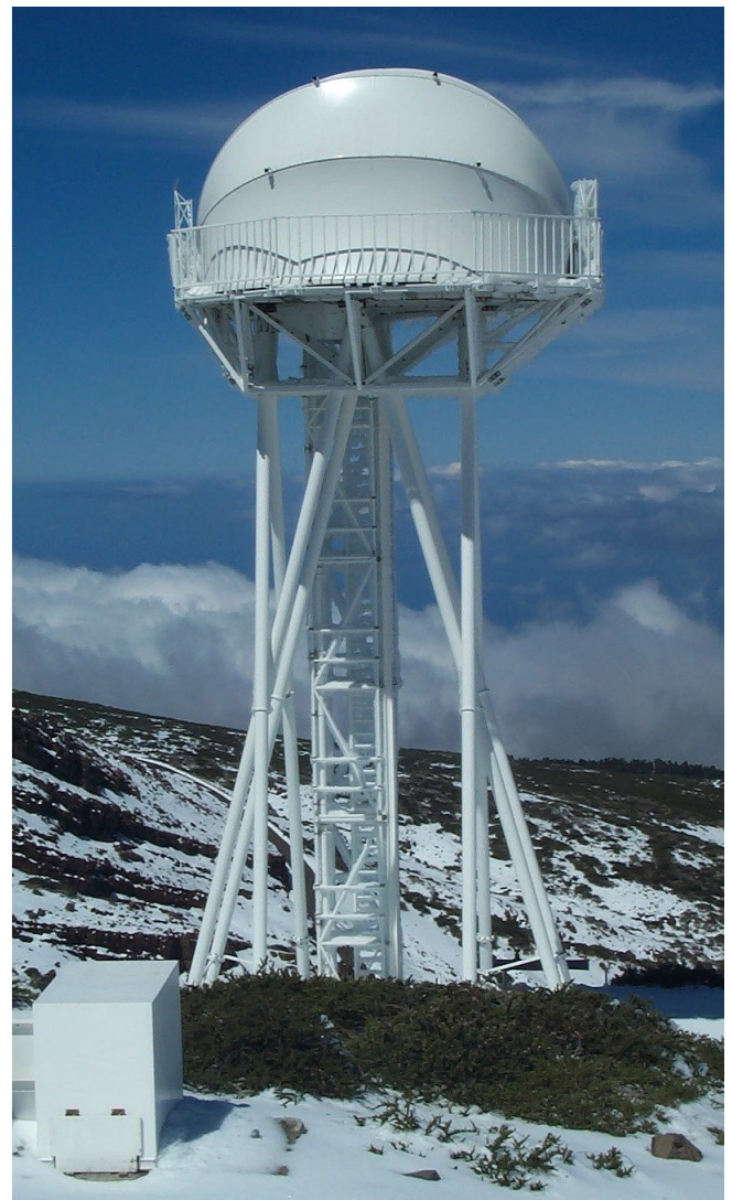
Figure 2. The DOT on its open steel framework tower with a height of 15m. The left picture shows the enclosure open while the DOT is observing. The right picture shows the enclosure closed as protection against bad weather.
