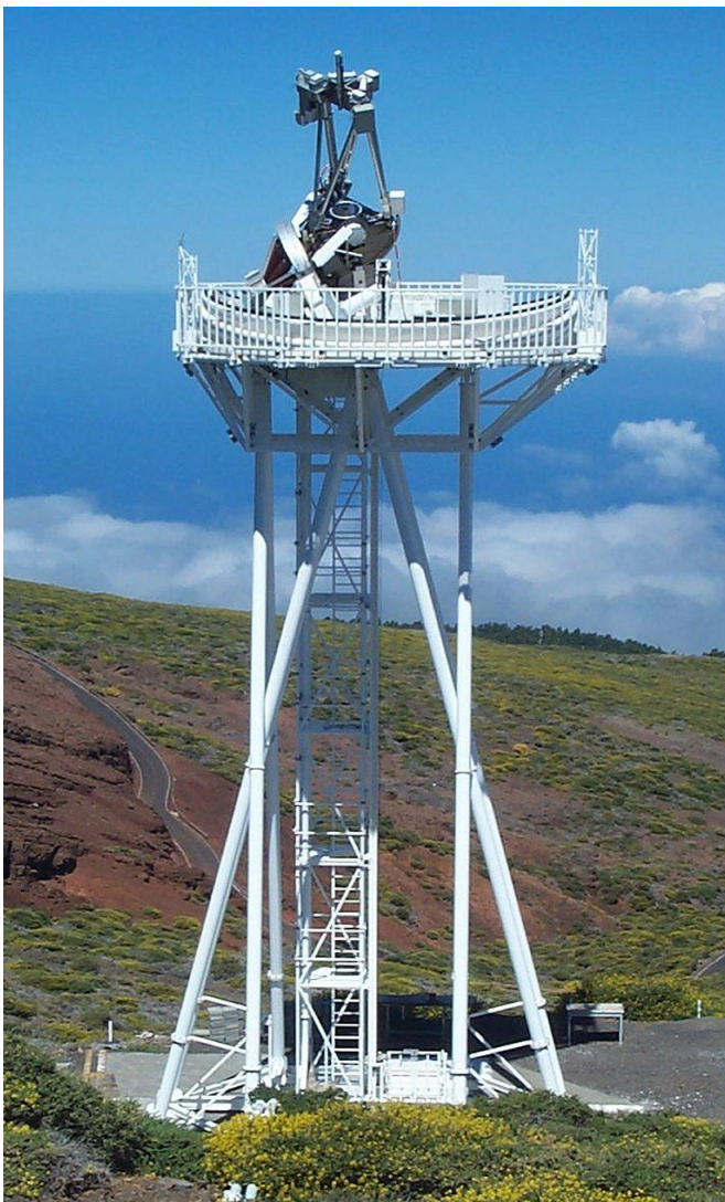
Figure 2. The DOT on its open steel framework tower with a height of 15m. The left picture shows the enclosure open while the DOT is observing. The right picture shows the enclosure closed as protection against bad weather.
